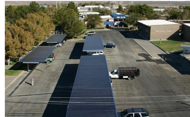
Naval Air Weapons Station – China Lake Solar carport (116 KW)
